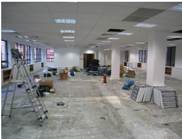
Photo – Works in progress to mitigate excessive landlord's claim
